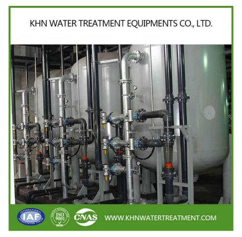
Quartz sand filtration is one of the most effective means to remove suspended solids in water. It is an important unit in advanced sewage treatment, sewage reuse and water supply treatment. Its function is to further KHN water treatment Co.,Ltd. http://www.khnwatertreatment.com
