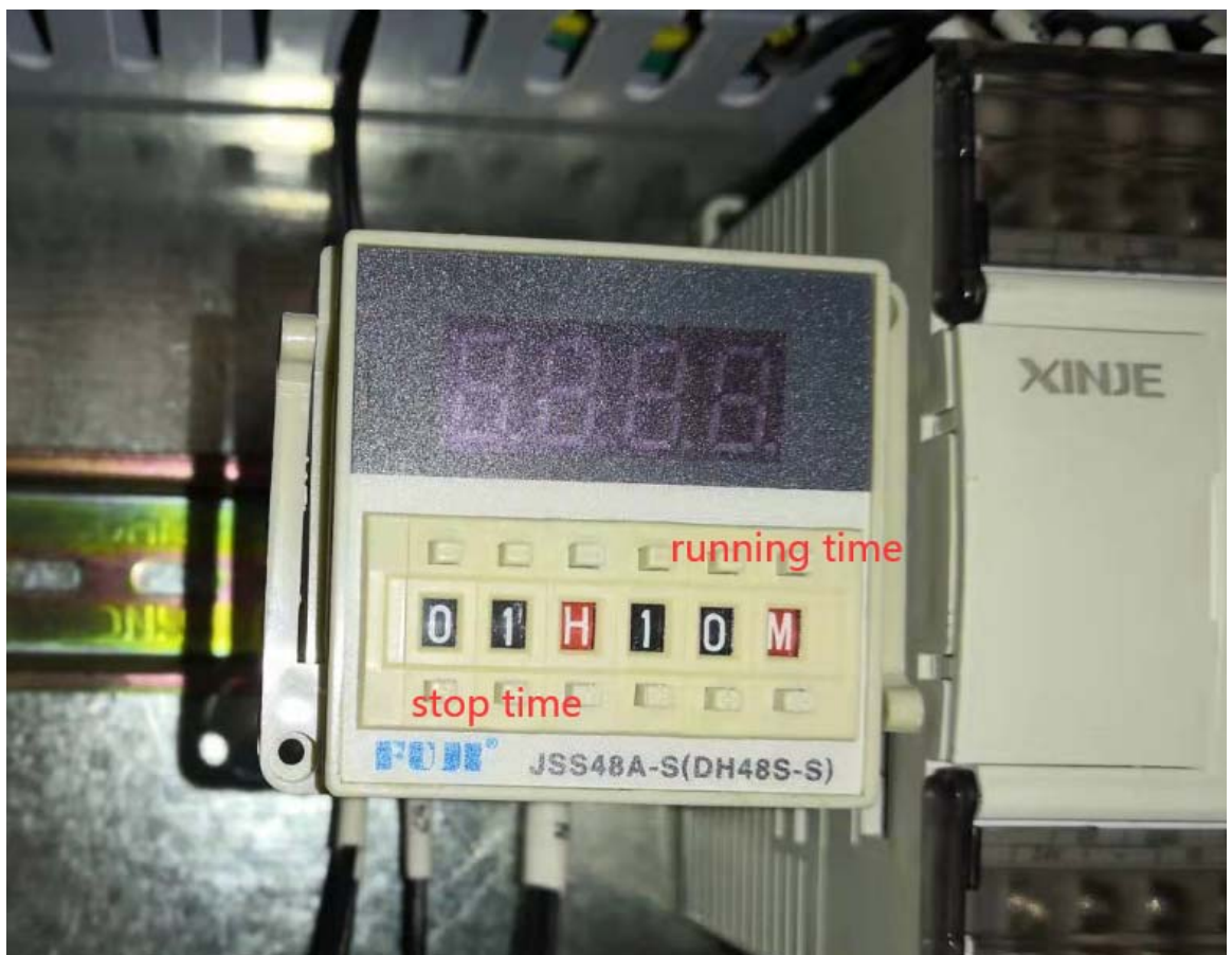
5.6 Slag scraper time adjustment
