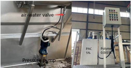
It is equipped to add flocculants PAC and Polymer to the dosing box, and the proportion of the prepared agent is 5% for PAC and 0.001% for Polymer.
